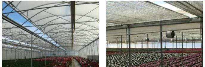
Roof and side ventilation, combined with the use of booster fans to create the largest possible air movement.
